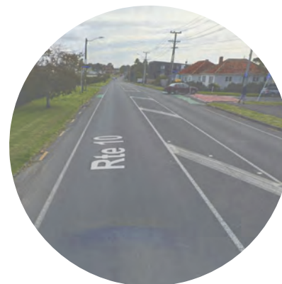
Carrington Road (Existing)
